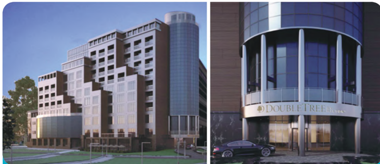
Double Tree(Hilton) in Russia, with 3-pipe VRF system.
