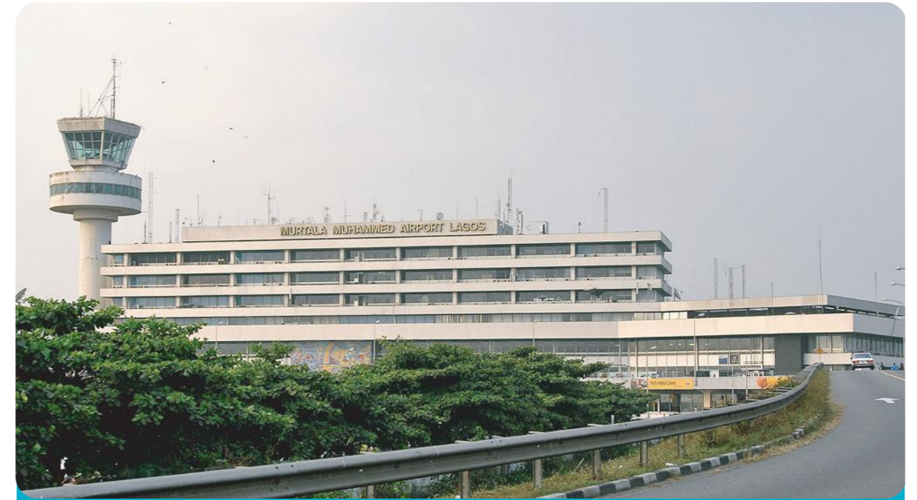
Murtala Muhammed Airport Lagos , total VRF capacity 800KW.
